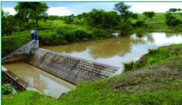
fig-1: Communitybased masonry dam
