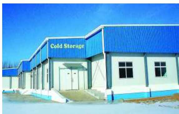
Fig-22 Cold storage unit
