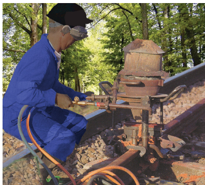
Figure 3.11 Thermit process for joining railway tracks
