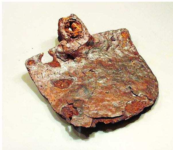
fig-15: Rusting of iron
