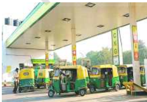
Fig - 3 CNG gas filling station
