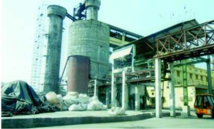
Fig 11.6 Pulping machine (Fiber line)
