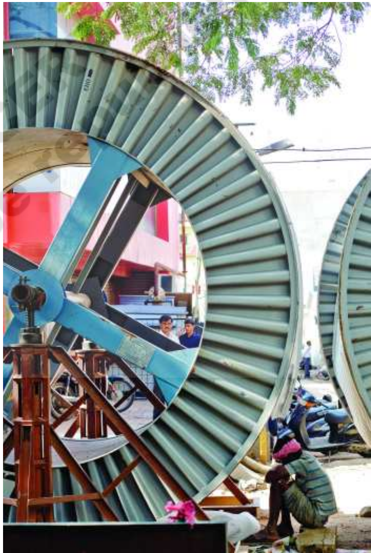
Fig 21.4 Workers laying cables
