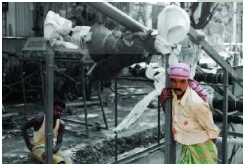
Fig 21.5 Road Laying Work
