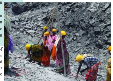
Fig 6.11: Women drilling holes for blasting
